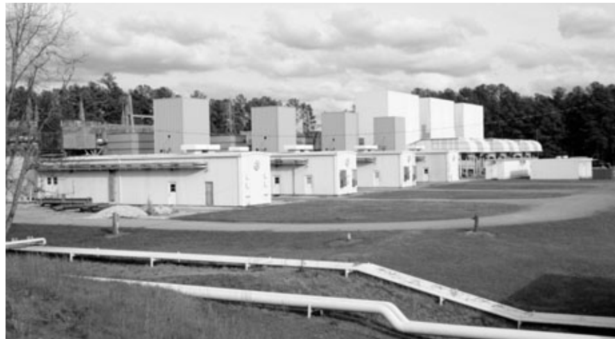
Combustion Turbine Installation
